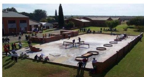
Large outdoor practical fire facility
